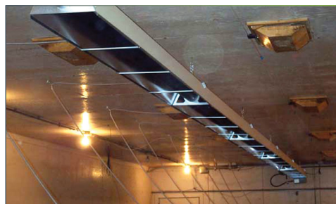
Figure 4. Typical infrared heater Source: Prairie Swine Centre
