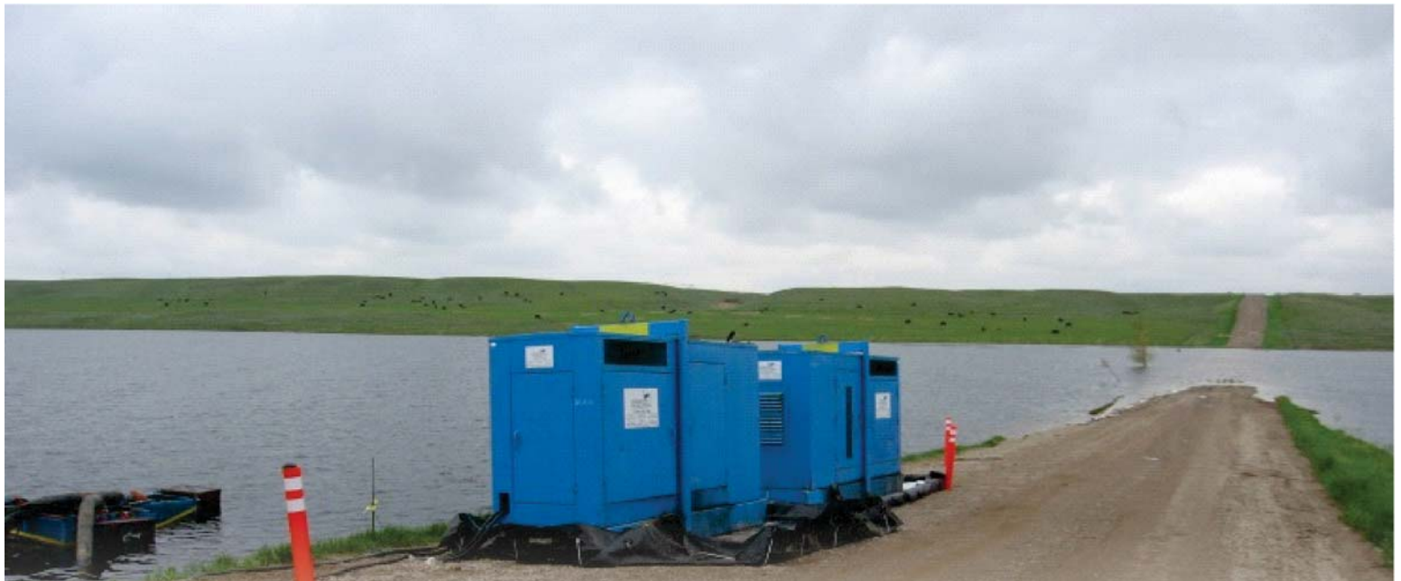
Flooding of road across Yellow Lake (2010).
