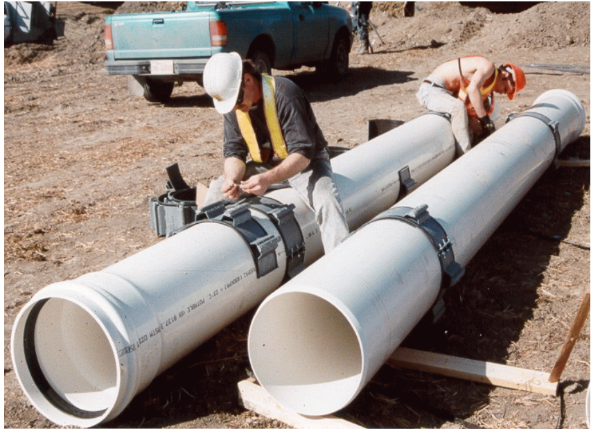
Casing spacers being installed on pvc pipe
