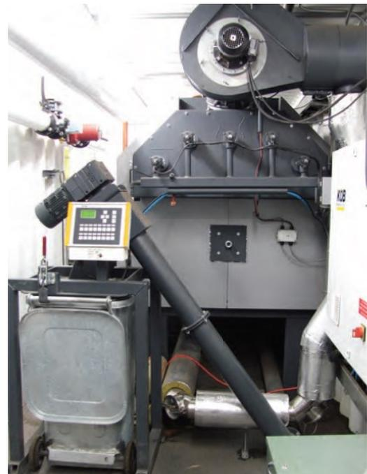
Figure 16: Lilloet 400kW pellet boiler, with ash auger and ash bin in foreground. Source: Green Energy as a Rural Economic Development Tool Project, D. Dubois, Case Study: District of Lilloet - Biomass Heating System, p.9
