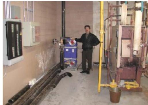
Figure 4: Energy transfer station in an old boiler room. Source: T. Berry, *Compass Resource Management, District Energy Primer, 2012, p5.*
