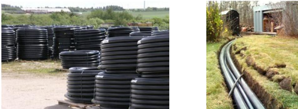
Figure 18: Left – rolls of insulated PEX pipe, with bonded insulation and bonded jacket. Right – insulated PEX pipe in a trench, prior to backfilling. Source: Urecon.
