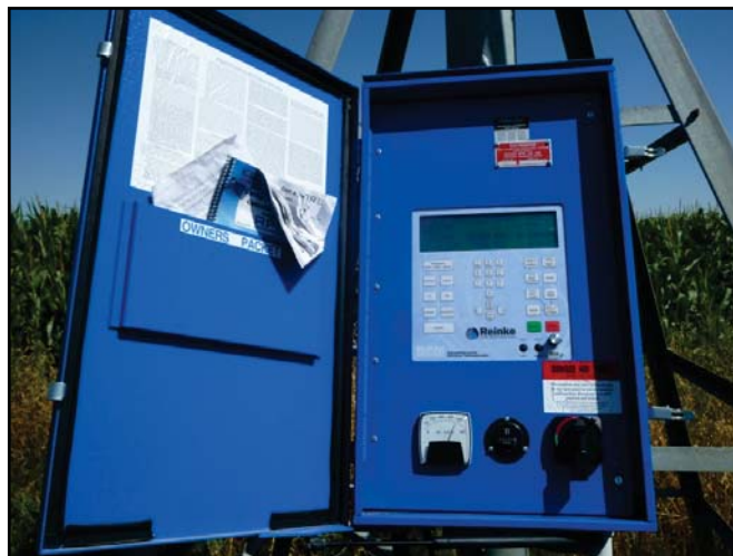
Figure 5.4. Control panel installed on the pivot irrigation system at the Battersea Drain Field in August 2012.
