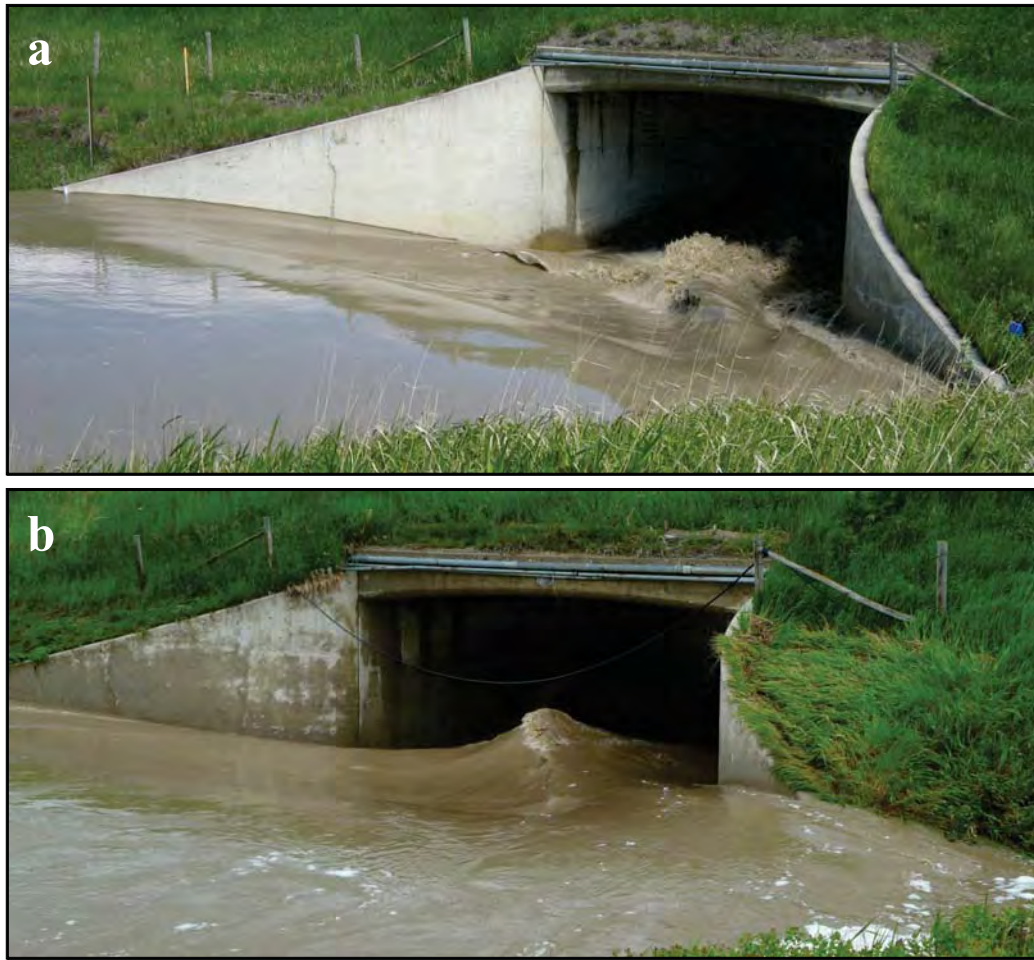
Figure 3.18. The outlet on (a) June 12, 2008 and (b) June 17, 2010. The difference in flow between the two dates can be seen at the sides of the concrete structure of the road bridge.
