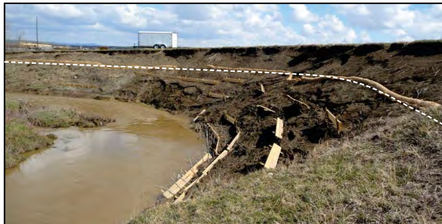
Figure 3.75. Damage to the bioengineering structures installed in April 2010. The dotted line shows approximately the high water level during peak flow.
