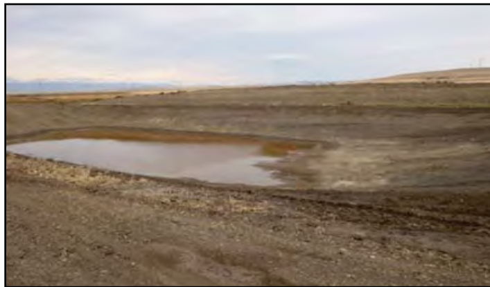
Figure 3.140. A new catch basin was established northeast of existing feedlot to receive runoff from the new feeding and bedding area. Image was taken October 21, 2011.
