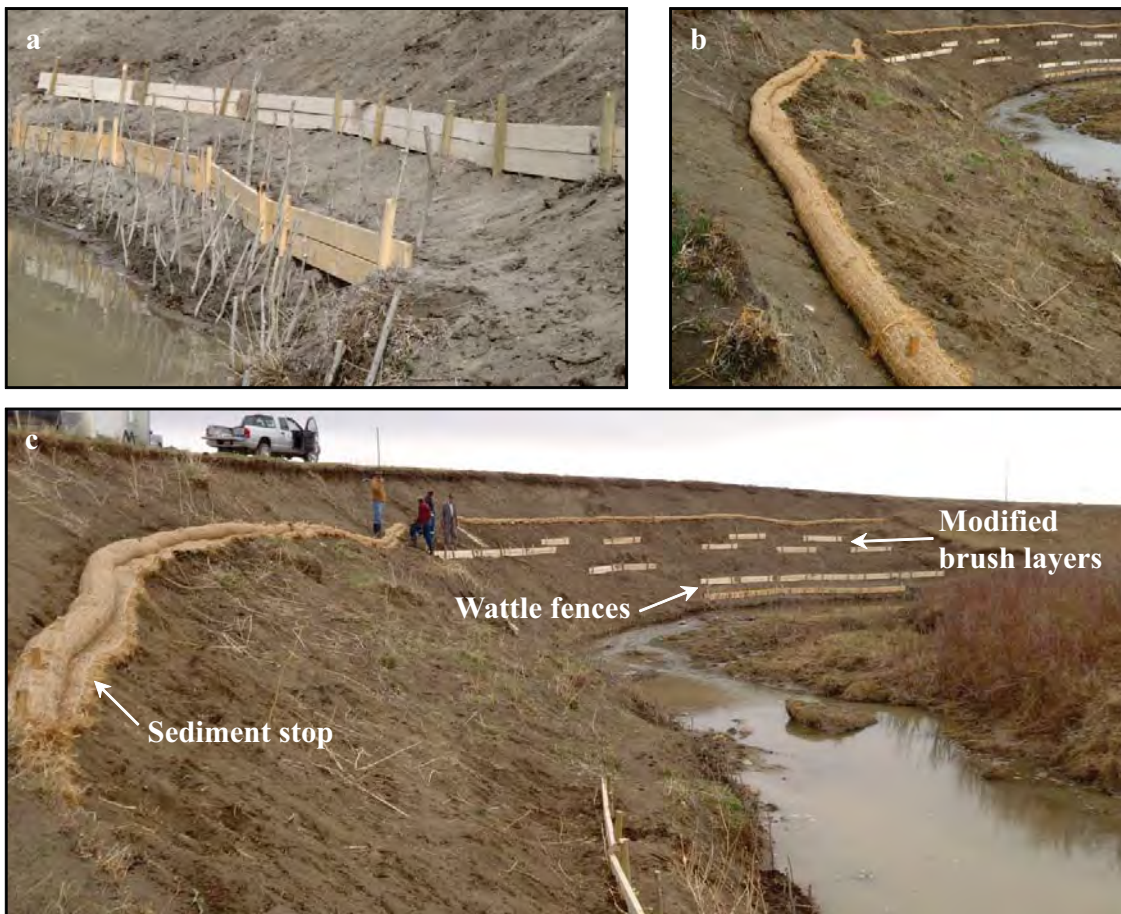
Figure 3.71. Bioengineering installation at the Pasture site showing (a) wattle fence, (b) sediment trap and modified brush layers, and (c) the whole bioengineered site on April 26 and 27, 2010.
