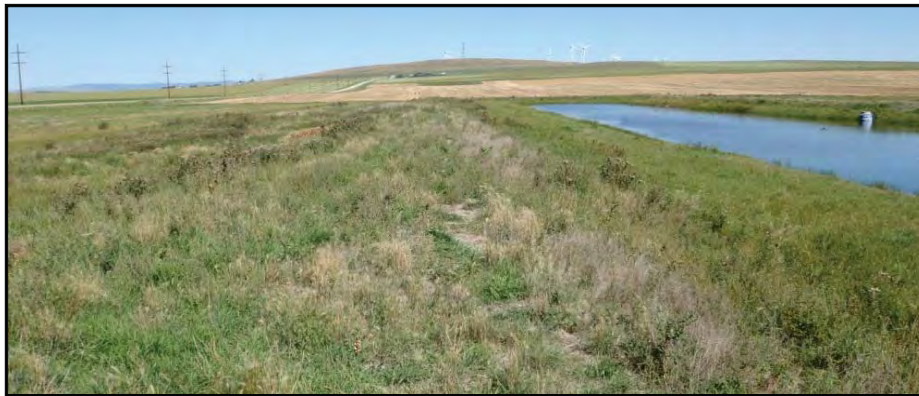
Figure 3.142. Vegetation growth on the berm along the west side of the dugout at the Feedlot site on August 21, 2013.
