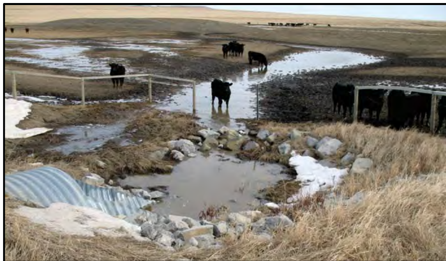
Figure 3.137. Cattle in the tributary at the Feedlot site as viewed near Station 24 where water from the tributary flowed through culverts under the road. Image was taken on March 3, 2010.
