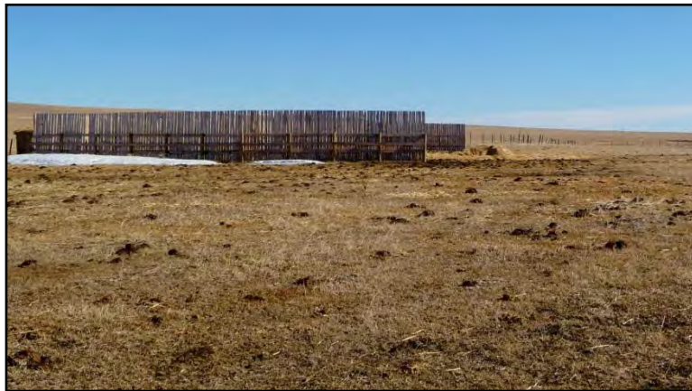
Figure 3.86. The wintering bedding and feeding site constructed in 2008.
