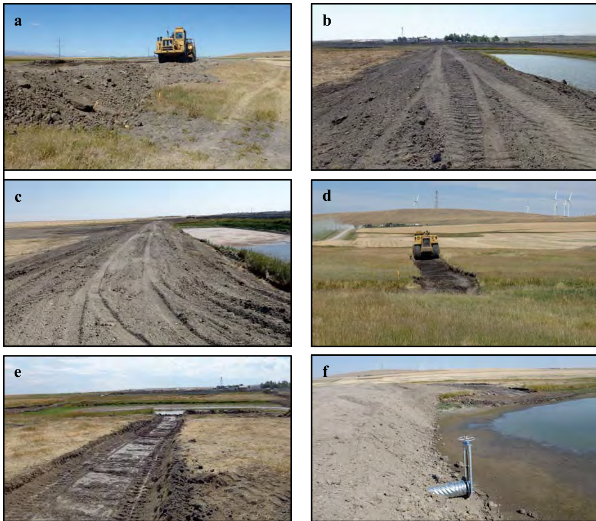
Figure 3.139. Construction activities at the Feedlot site showing the new berms on the (a) west side and (b) east side of the dugout. Also showing (c) the berm on the north side of the catch basin, (d) the new diversion channel along the west side of the dugout, (e) the diversion channel exiting the north side of the settling pond, and (f) the sluice gate installed between the dugout and settling pond. Images were taken August 24 to September 12, 2011.
