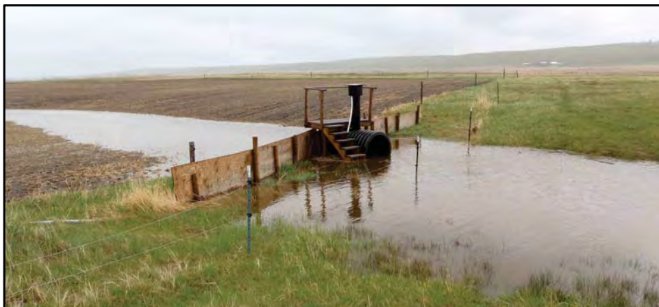
Figure 3.114. Station 21 flooded with backed up water from the tributary on May 24, 2011.
