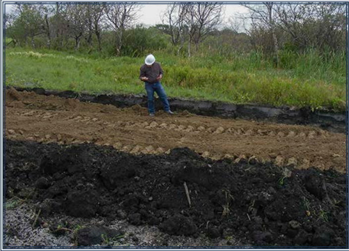
Holding pond construction.
