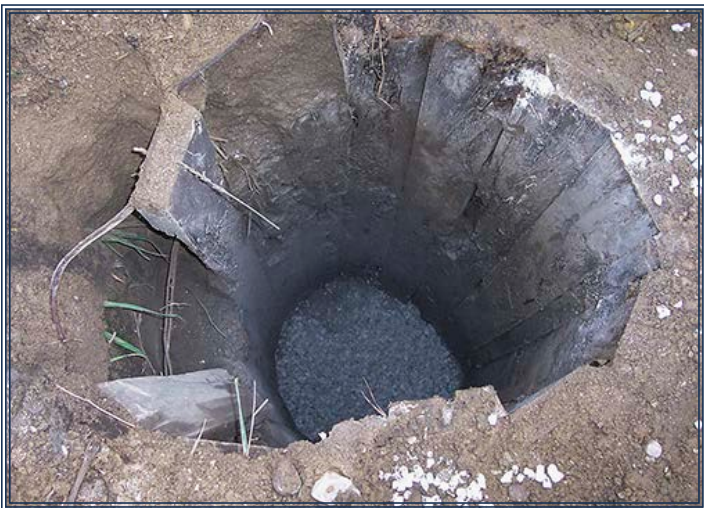
Bentonite seal in a decommissioned well.
