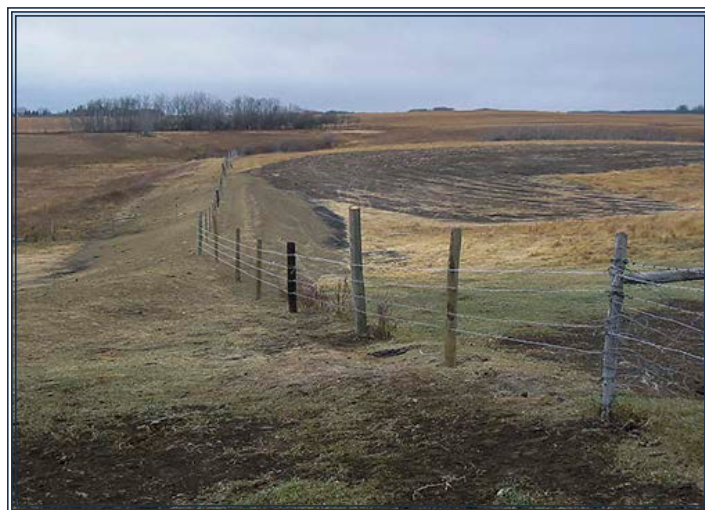
Berm to direct runoff water.
