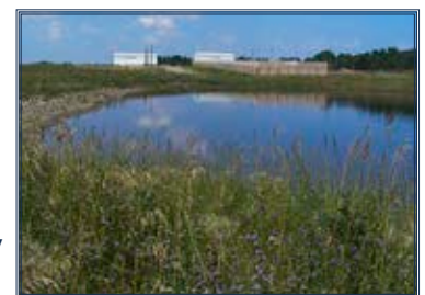
Holding pond for control of runoff.
