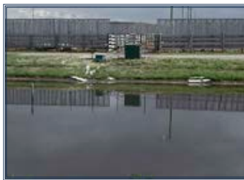
Runoff control structures can be implemented to minimize environmental risks
