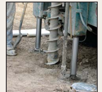
Auger drilling
