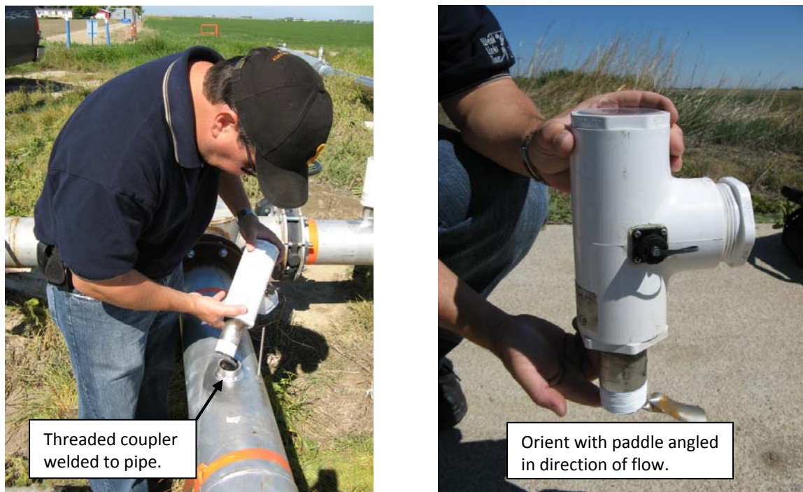
Figure 3. Installing the model LOPAC LHE2 monitor.
