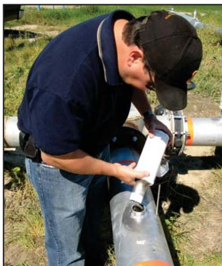
**Installing LOPAC into threaded coupler welded to pipe**
