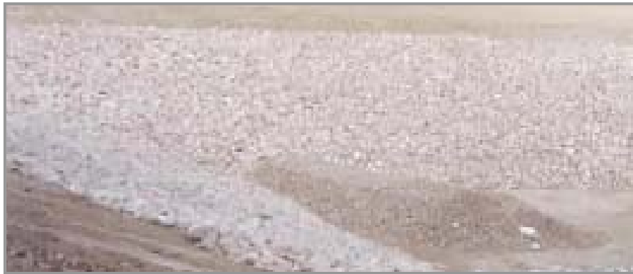
Gabion Wall Infiltration System - Empty
