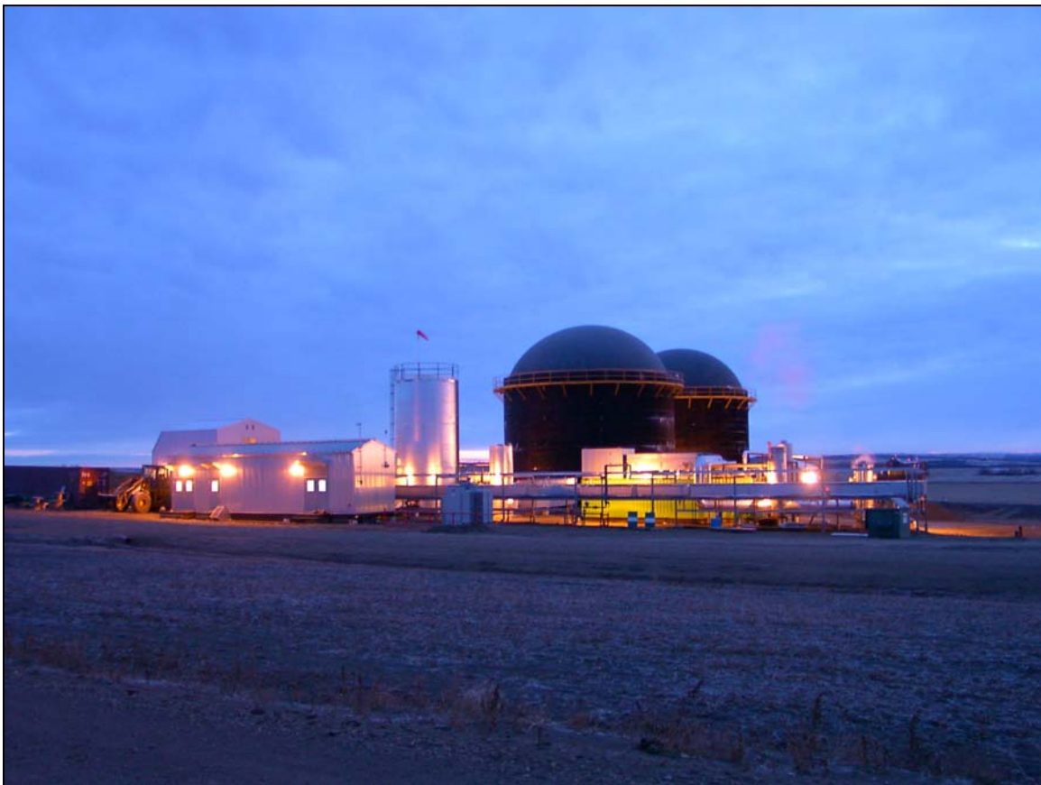
Biodigester – Highland Feeders, Alberta
