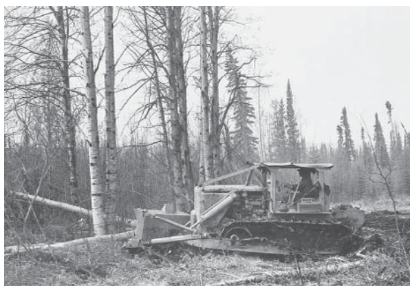
Building the Forestry Trunk Road, Mist Creek, Bow River Forest, 1951 Alberta Government, AFHPC
