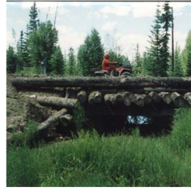
Figure 49. Native Timber Bridge
