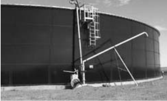
Figure 10. Above ground concrete liquid manure storage that can be used in places where soil conditions would pose risk to drinking water if earthen storages were used. Source: Kai Ma, NRCB.
