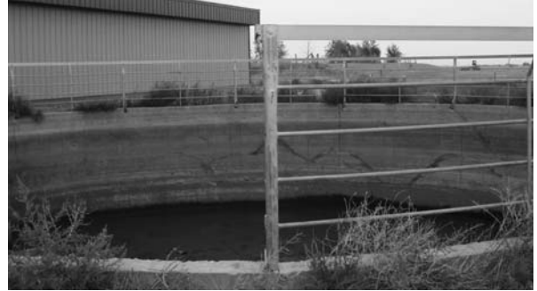
Figure 11. A concrete liquid manure storage tank with chain link safety fence. Source: Matt Oryschak, AAFRD.
