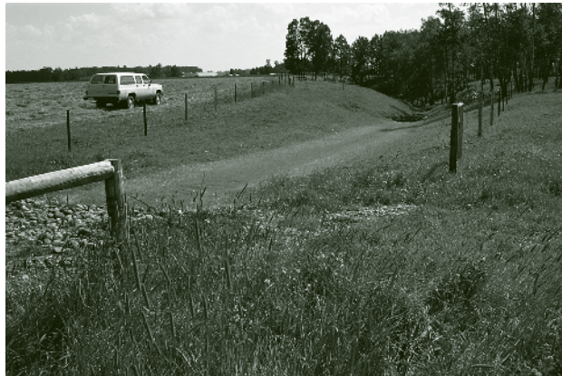
Figure 8.3.3 Constructing Grassed Waterways.
