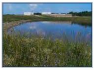
Holding pond for control of runoff.
