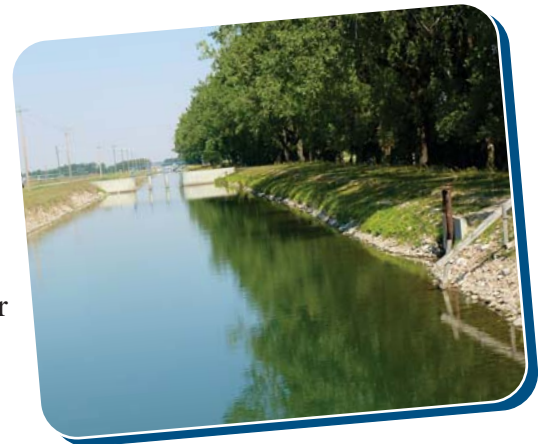
Water Supply Canal
