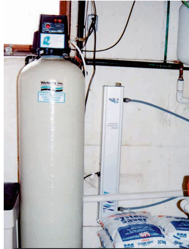
An add-on softener will reduce hardness. The ultraviolet light (UV) was added after the softener to disinfect the ground water
