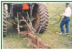
Shallow ploughed installation of pasture pipeline
