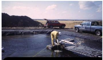
A cell is coagulated by pouring the chemical in the water near the trolling motor
