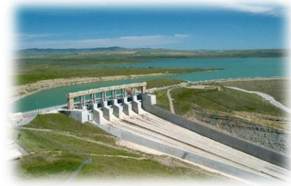
Oldman dam and reservoir
