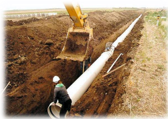
Installation of a district pipeline
