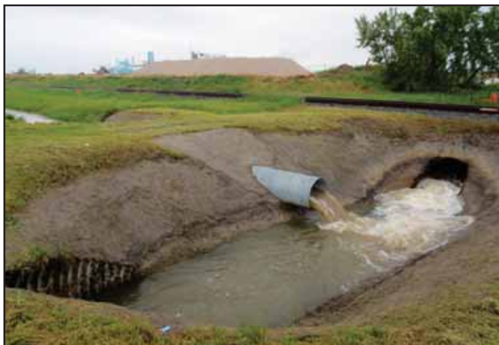
Drain inlet site T-LU3 draining municipal stormwater into an irrigation canal of TID.
