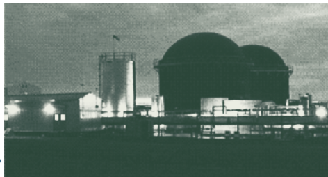
Anaerobic digester and energy cogeneration plant near Vegreville
