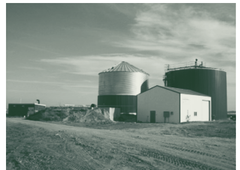
Anaerobic digester and energy cogeneration system near Cudworth, Saskatchewan
