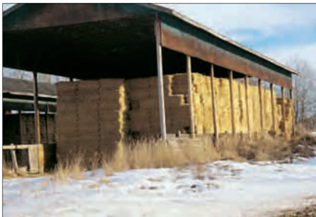
HAY SHED USED TO REDUCE WEATHERING LOSSES
