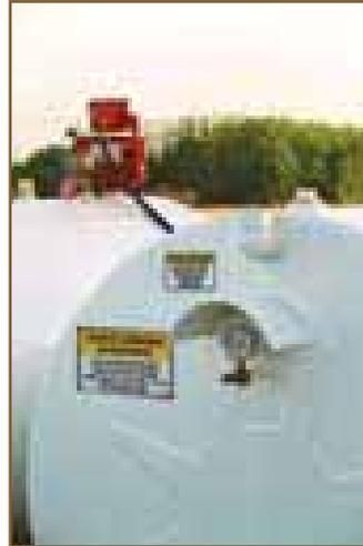
*Figure 12: Double wall vacuum monitoring gauge
