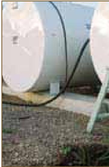
*Figure 17: Double walled tanks using concrete supports on firm, compacted gravel
