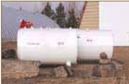
*Figure 18: Collision protection using large boulders
