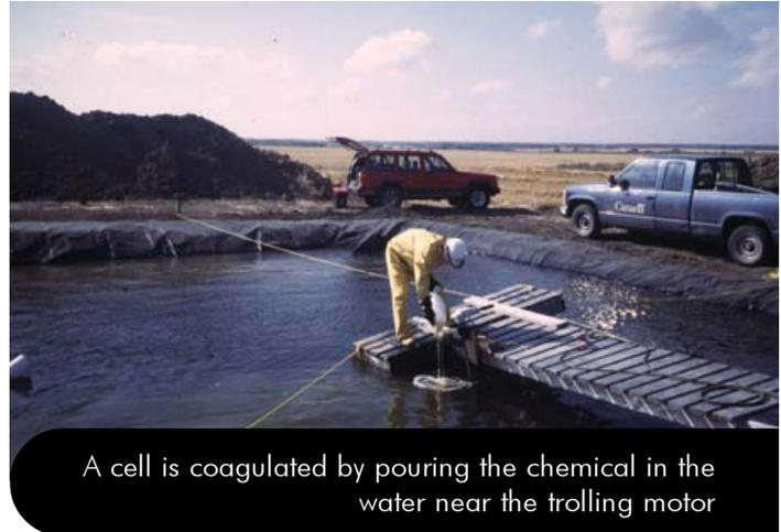
A cell is coagulated by pouring the chemical in the water near the trolling motor
