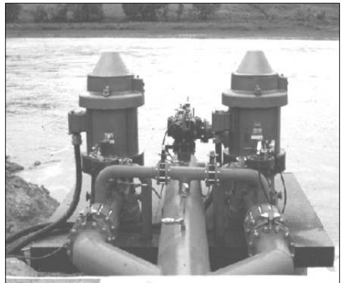
A typical fixed pump site.
