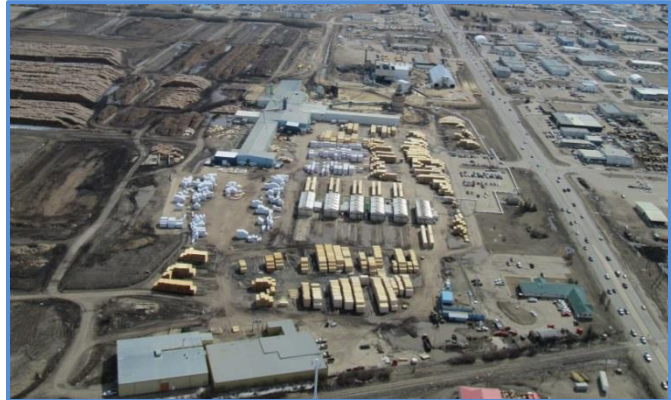
Figure 2 Canfor Grande Prairie Sawmill and Co-generation Facilities
