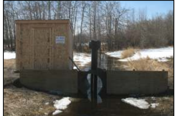
Water monitoring station
