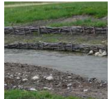
Lyndon Creek bioengineering project
