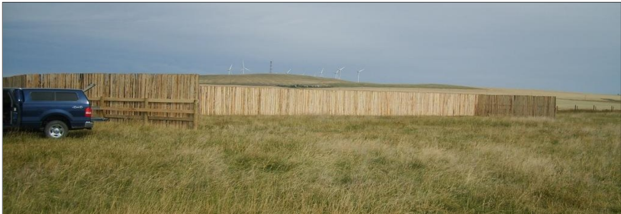
Construction of a new wintering site.
