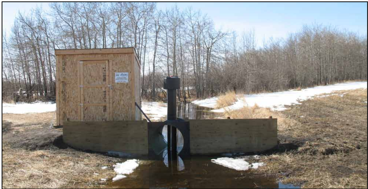
Water monitoring station in the Whelp Creek Sub-watershed showing a circular flume and equipment shed.
