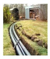
Figure 18: Left – rolls of insulated PEX pipe, with bonded insulation and bonded jacket. Right – insulated PEX pipe in a trench, prior to backfilling. Source: Urecon.
