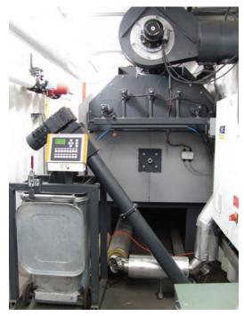
Figure 16: Lillooet 400kW pellet boiler, with ash auger and ash bin in foreground. Source: Green Energy as a Rural Economic Development Tool Project, D. Dubois, Case Study: *District of Lillooet - Biomass Heating System*, p.9
