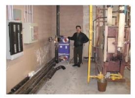
Figure 4: Energy transfer station in an old boiler room. Source: T. Berry, Compass Resource Management, *District Energy Primer*, 2012, p5.
