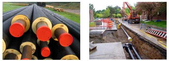
Figure 17: Left – thin-walled steel carrier pipe with bonded hard polyurethane insulation, built-in leak detection system, and bonded high-density polyethylene outer jacket. Right – insulated steel pipe being lowered into place in a trench. Source: Natural Resources Canada and FVB Energy via Canadian District Energy Association *Biomass for District Heating* module.
