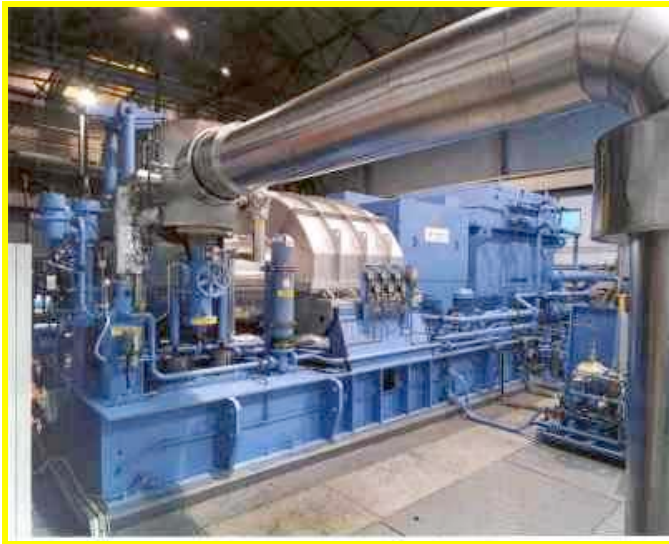
Section through a steam turbine above. Condensation steam turbine with 10 MWe below. Source: Energytech 31
