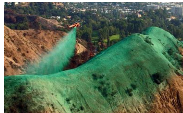
Synermulch Erosion Control Products Inc. - Hydro seeded flax erosion control product
