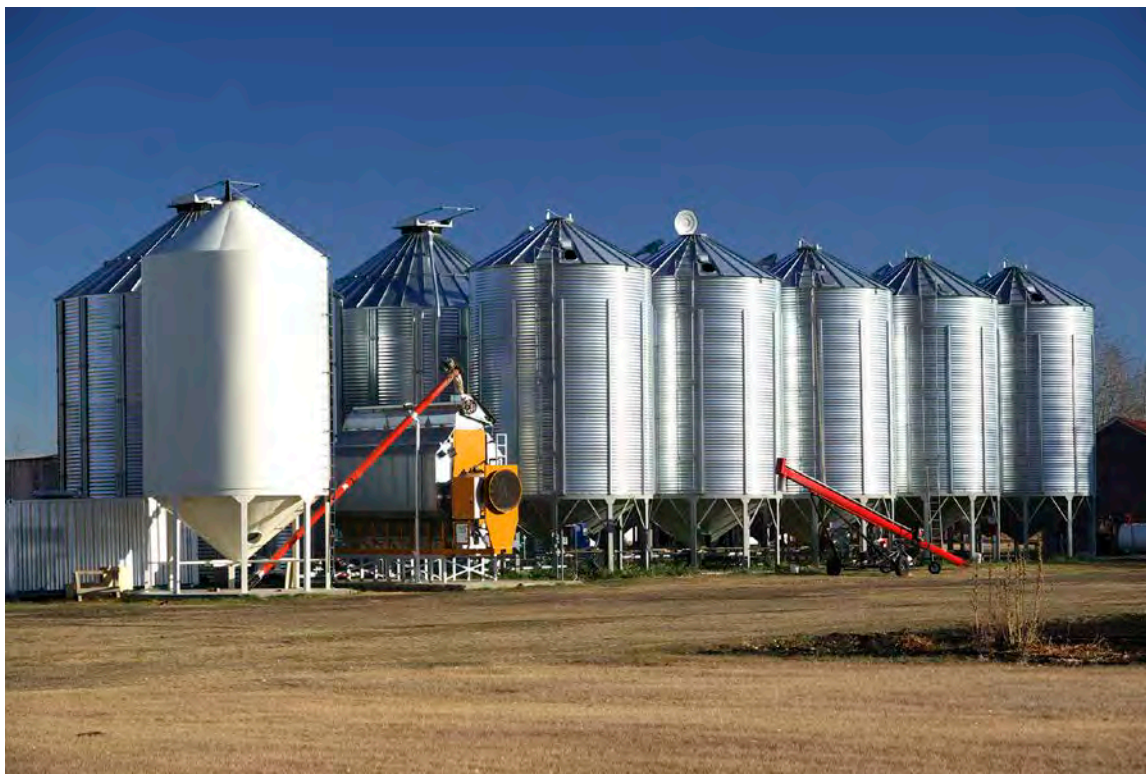
Photo 11: Hopper bin with aeration and grain dryer
