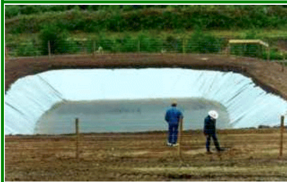
Raised earthen storage with woven polyethylene liner Source: Pasture Water Systems for Livestock, Alberta Agriculture, Food and Rural Development, http://www.agric.gov.ab.ca/agdex/400/400_716-3.html
