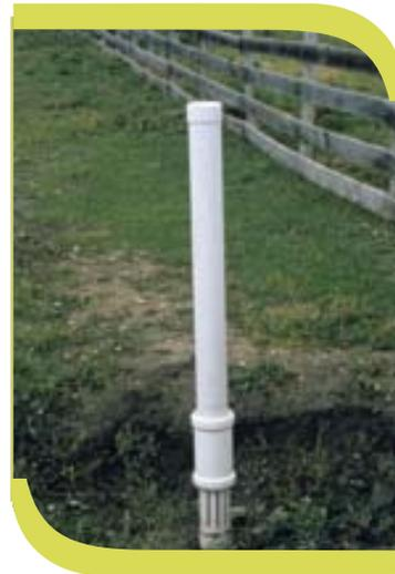
A clean water inlet pipe collects clean runon water upslope of a livestock yard and discharges it below the yard through a drain outlet.
