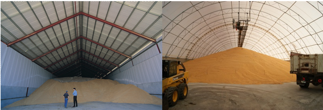
Figure 6. Grain Storage Sheds
