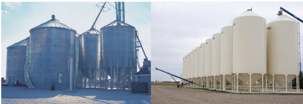
Figure 5. Steel Grain Bins (Corrugated and Smooth Walled)
