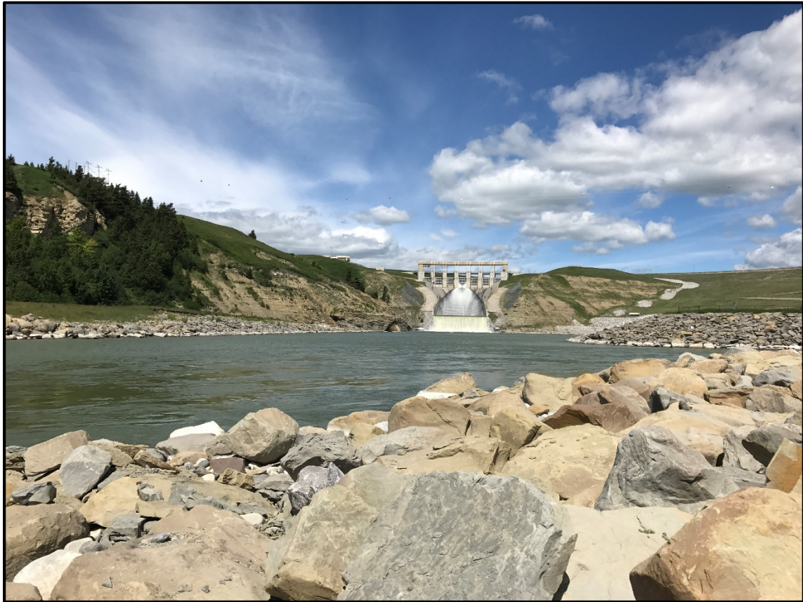
Spillway of Oldman River Dam and Reservoir
