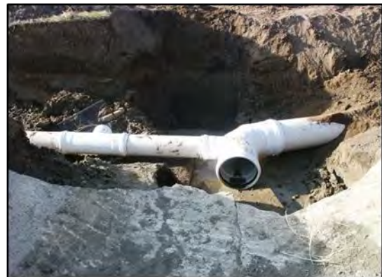
Pipe size reduction junction
