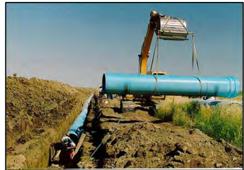
Underground irrigation pipeline installation
