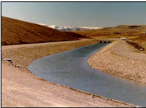
Armoured irrigation canal
