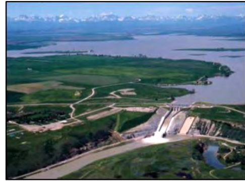
St. Mary Dam and Reservoir
