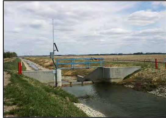
Water remaining in canal after fall drainage
