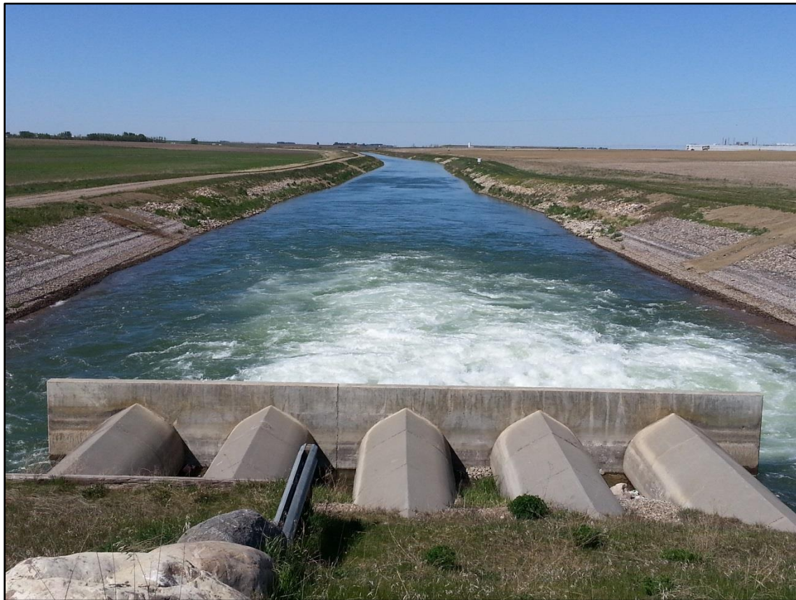
Outlet at north end of Stafford Reservoir
