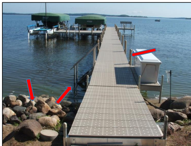
Figure 6. Inspection locations at a boat launch, including shoreline rocks, and dock railings and support stakes, as indicated by red arrows.
