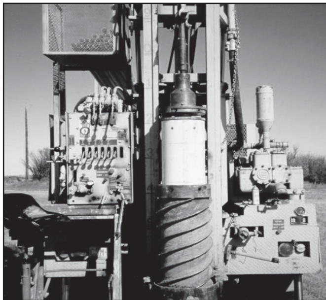
Figure 1. Drill truck with PVC pipe and hollow-cylinder.
