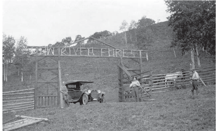
Construction near completion on new gateway into the Bow River Forest, c. 1915 Dominion Forestry Branch, AFHPC
