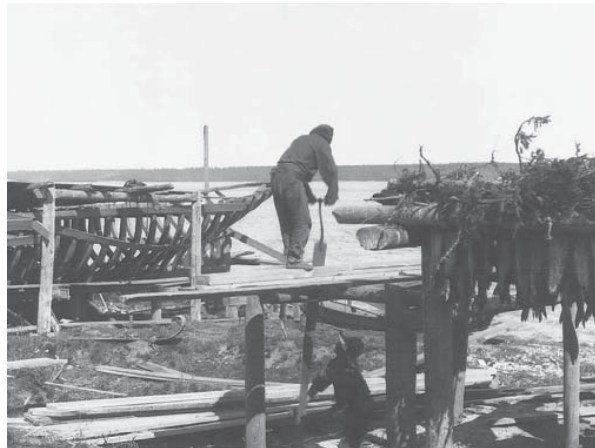
Pit-sawing lumber, Fort Smith, NWT, 1900 Provincial Archives of Alberta
