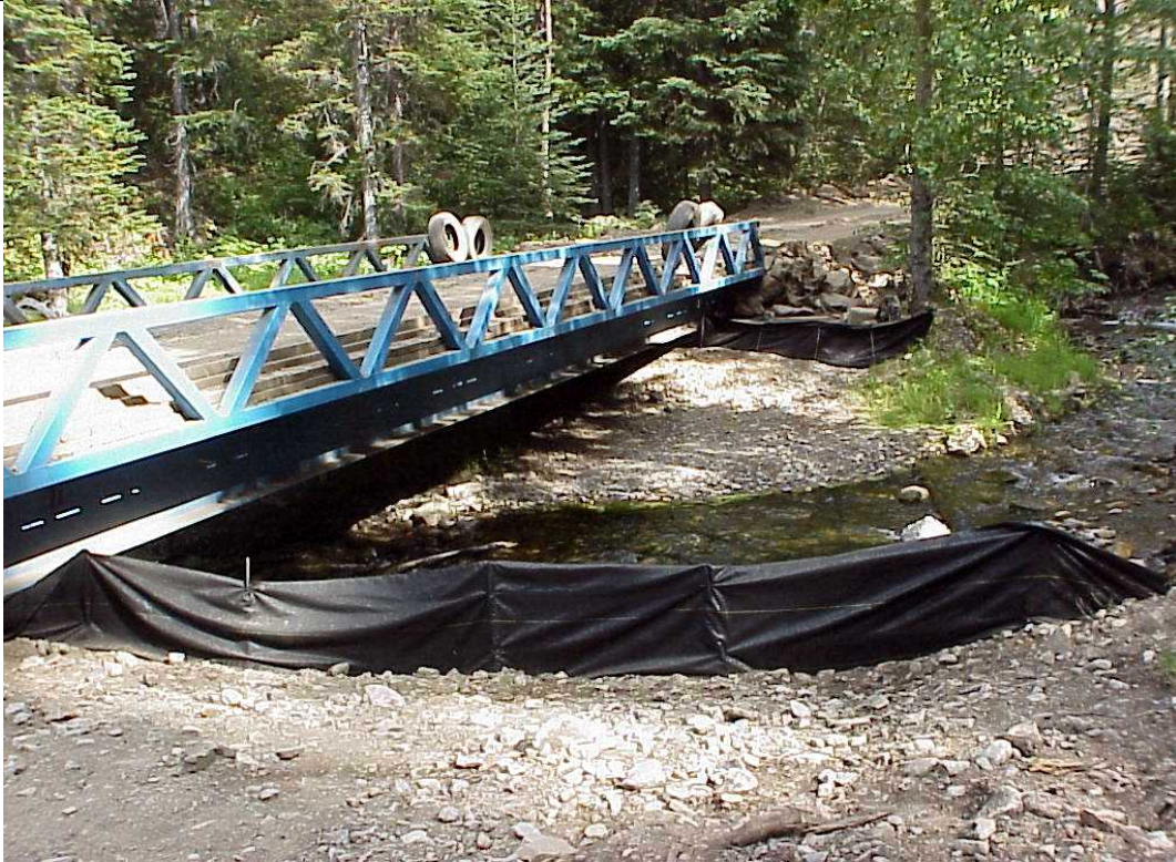
Proper temporary bridge installation will protect streams.
