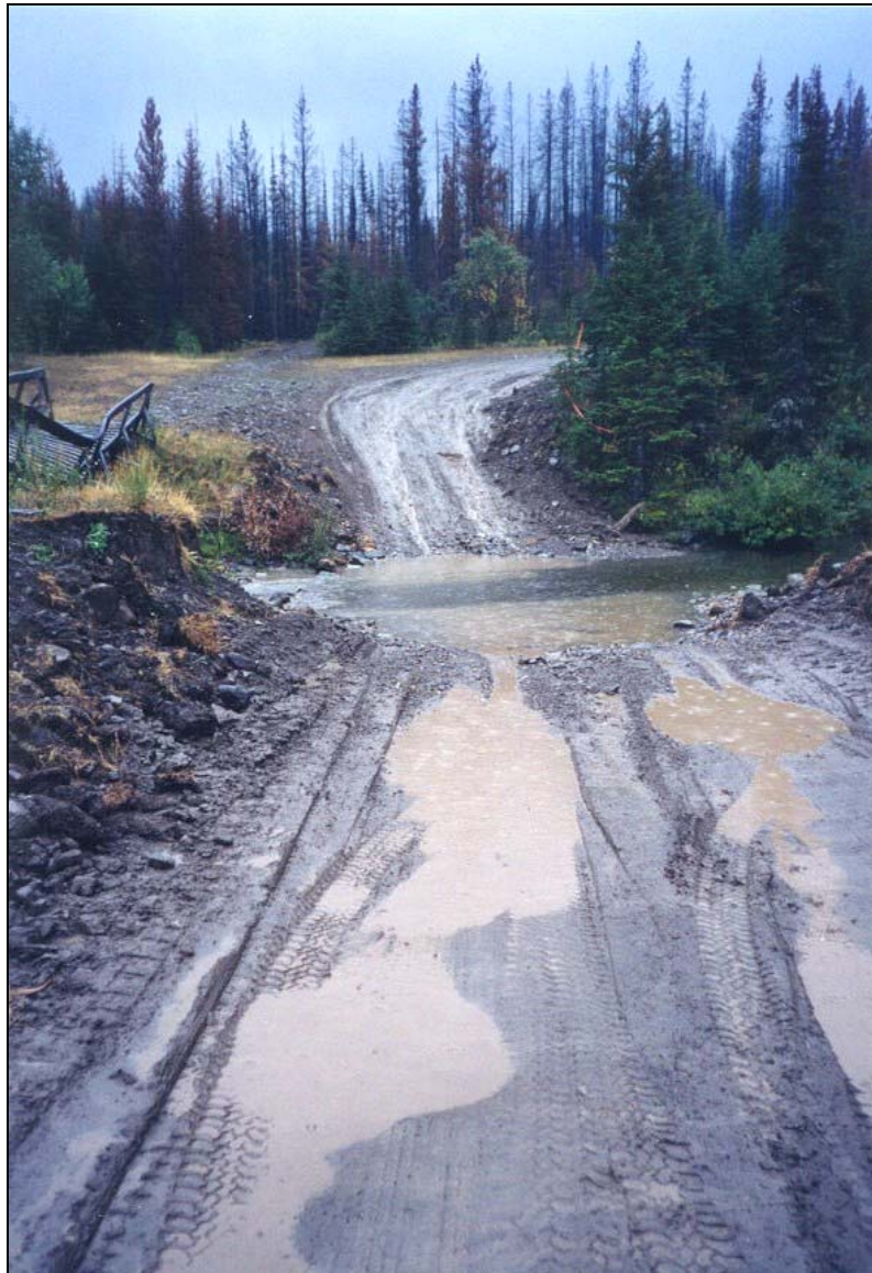
Temporary ford on South Lost Creek showing erosion.
