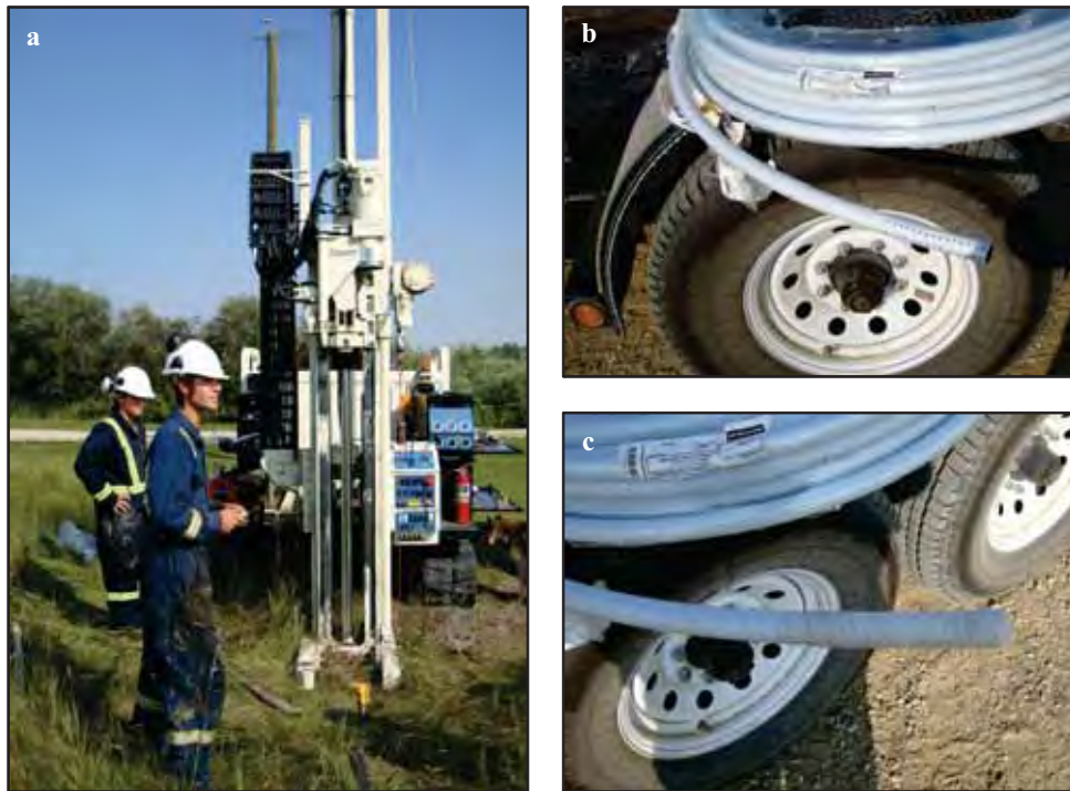
Figure 5.11. Installation of groundwater wells and piezometers.
