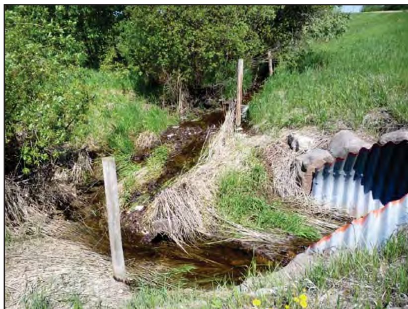
Figure 4.12. Station 303 was often influenced by water flowing through a road ditch from the north (top) and into the mainstem (flow from the left). Station 303 was located at the downstream end of this culvert (to the right). Image was taken June 12, 2010.
