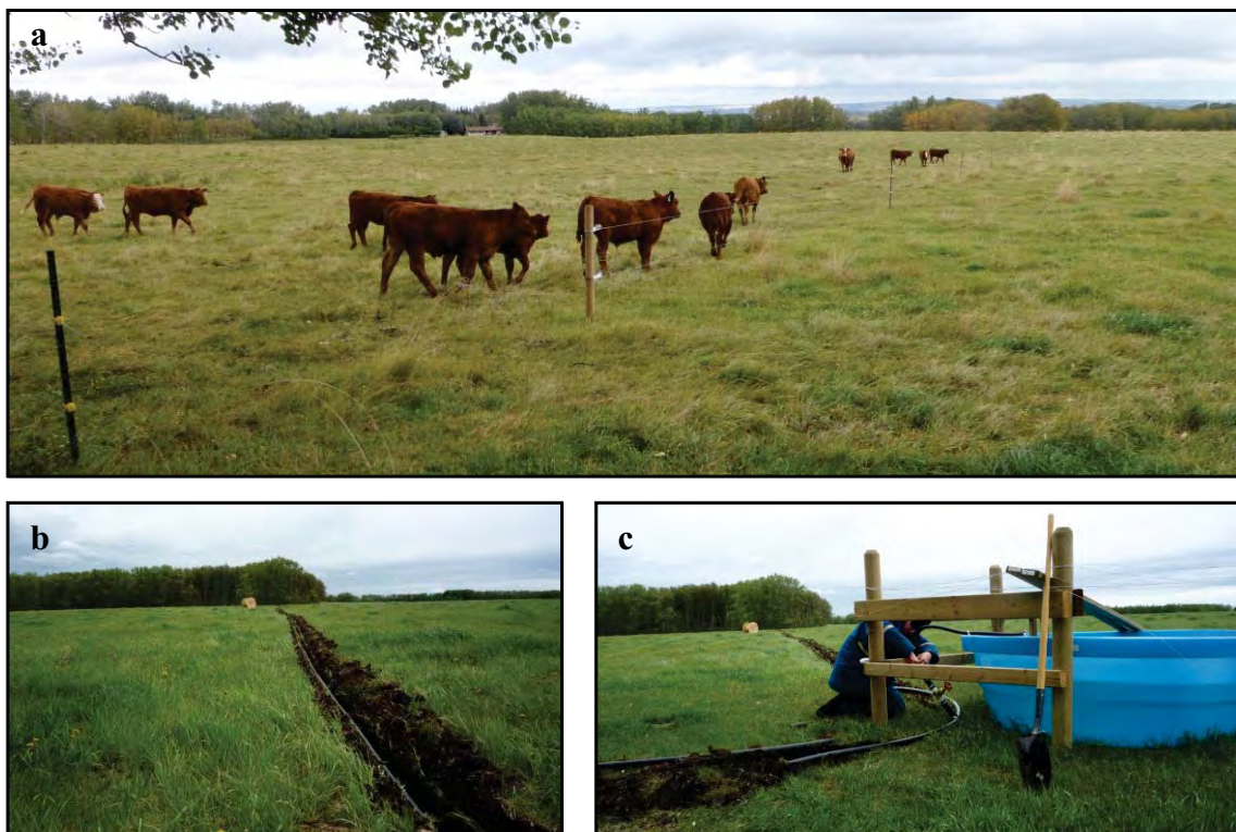
Figure 4.73. At the South Pasture, (a) electric fences was used to divide the pasture into paddocks and a (b) underground water pipeline and (c) water troughs were installed to supply water to the paddocks. Images taken on September 16 (top) and June 3 (bottom), 2010.
