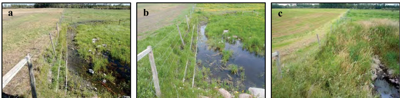
Figure 4.67. The bioengineering site on Whelp Creek at the North Pasture on (a) September 17, 2010 (about 1 mo after construction), (b) June 6, 2011, and (c) August 14, 2012.
