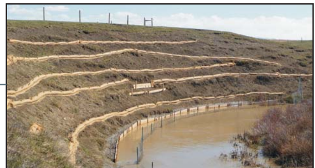
April 30 – live stakes were planted and a reclamation grass seed mixture was spread over the entire site – species used were red osier dogwood, willow, cottonwood and prickly rose
