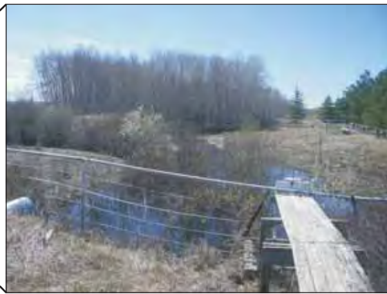
Whelp Creek diversion infrastructure
