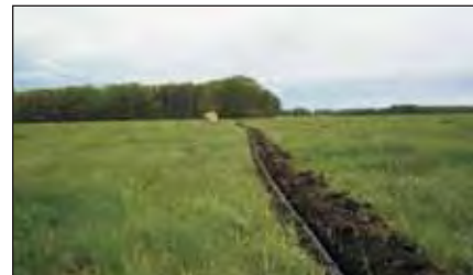
Water line installation
