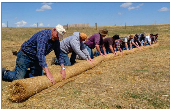
Figure 7.2. Learning how to prepare a sediment trap at the bioengineering field day held in April 2010 in the Indianfarm Creek Watershed.
